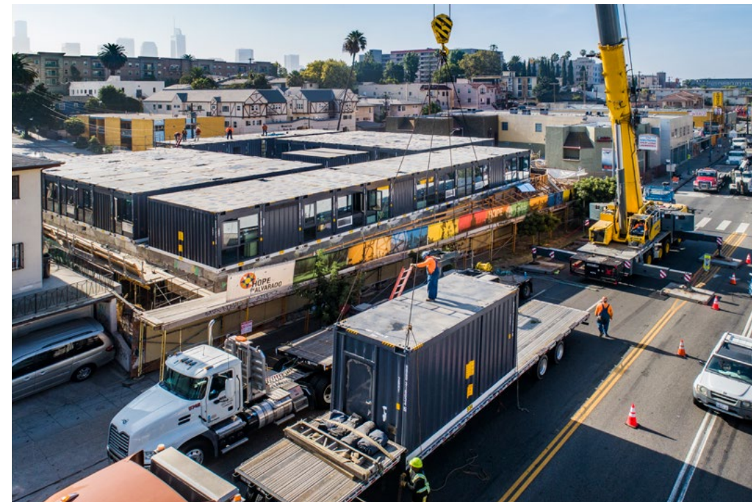
The steel modules for Hope on Alvarado were trucked to the site before being craned into place over a site-built concrete podium—a process that took one month to complete.
