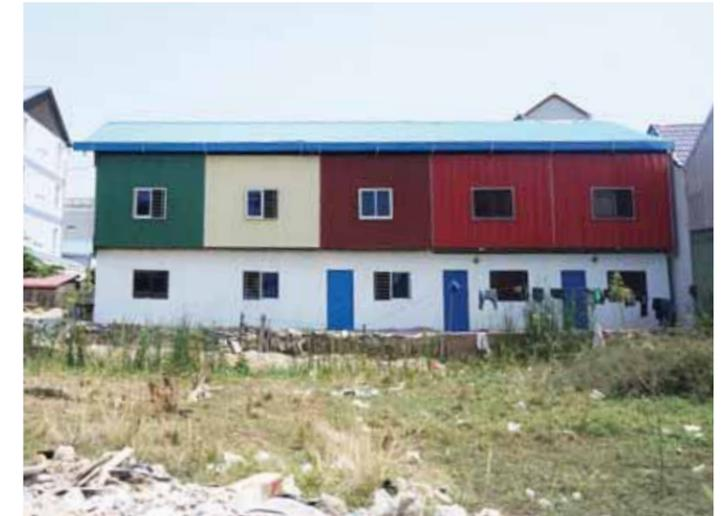
Seen typically in small groups or single strips, small scale townhomes are small family units that share side walls. When a lower height is maintained, natural ventilation is made possible through openings in the roof structure and front and back walls. By sharing side walls, these small units are able to conserve energy and also save construction materials.
