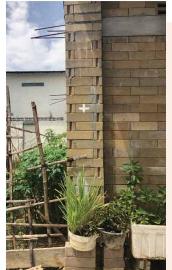
*Compressed earth blocks manufactured by HFH Cambodia used to construct HFH homes in Battambang.*
