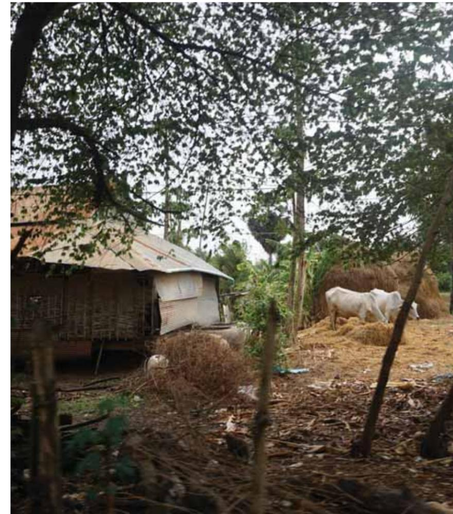
Village settlements are located outside of the city and typically occupied by multi-generational families. Village homes are constructed with a simple wood frame and consist of a variety of found and made materials. Some of these materials include: corrugated sheet metal, handmade sheathing and screens from fibrous vegetation, scrap construction material, and reusable products such as rice packaging.
