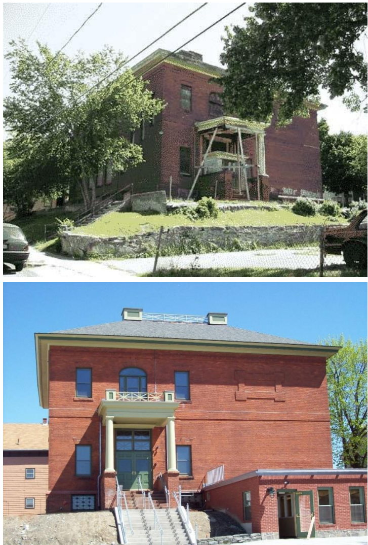
Figure 4: Hope Street Family Center, before renovation (top) and after renovation (bottom). Images courtesy of NeighborWorks Blackstone River Valley.
